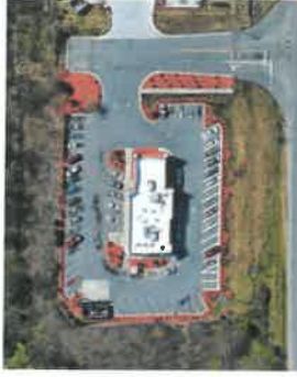
One-way angled parking facing the street can be used to reduce the building setback to approximately 30'
