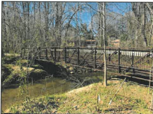
Sample pedestrian bridge
